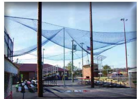
50603 Overhead Protective Netting
