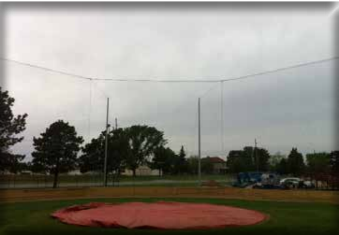
50601 Backstop Protective Netting
