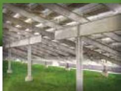
With I-beam understructure
