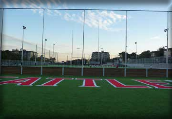
50601 Backstop Protective Netting
