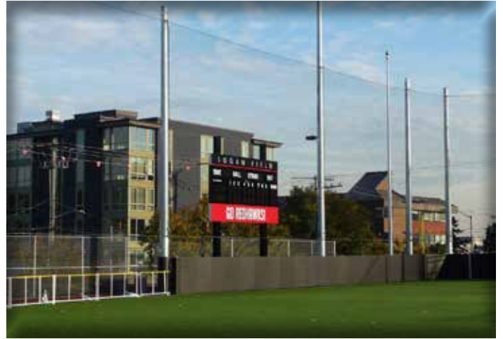
50602 Barrier Protective Netting
