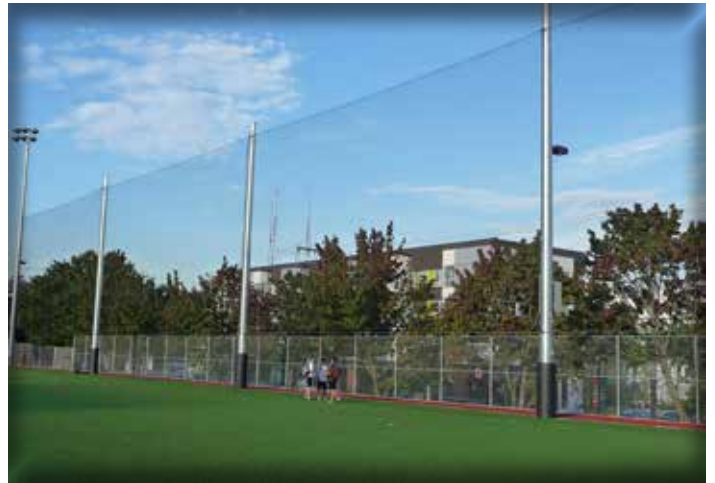
50602 Barrier Protective Netting
